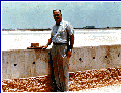
26" of concrete at Lubbock AFB in Texas.
